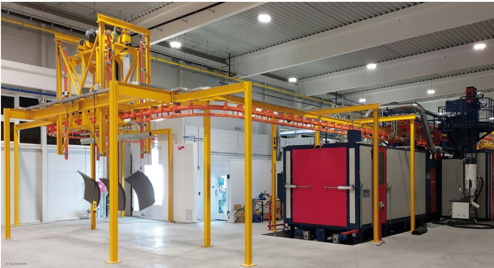
The liquid painting line with the automatic Power&Free overhead conveyor designed by Eurotherm.
