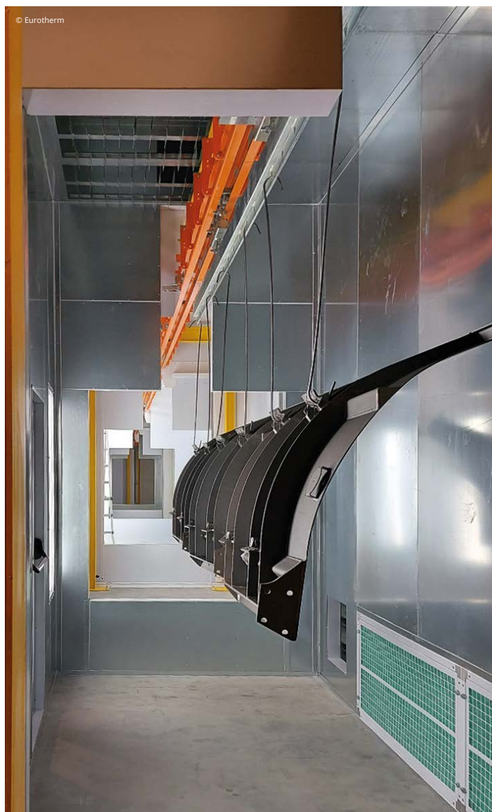
The flash-off tunnel.
