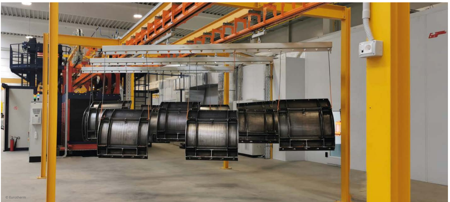
The automatic power&free overhead conveyor (on top) and the loading and unloading area.
