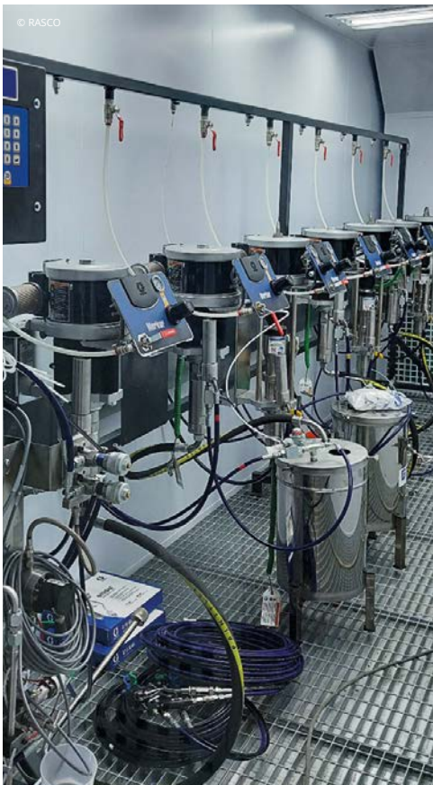
The paint kitchen.
